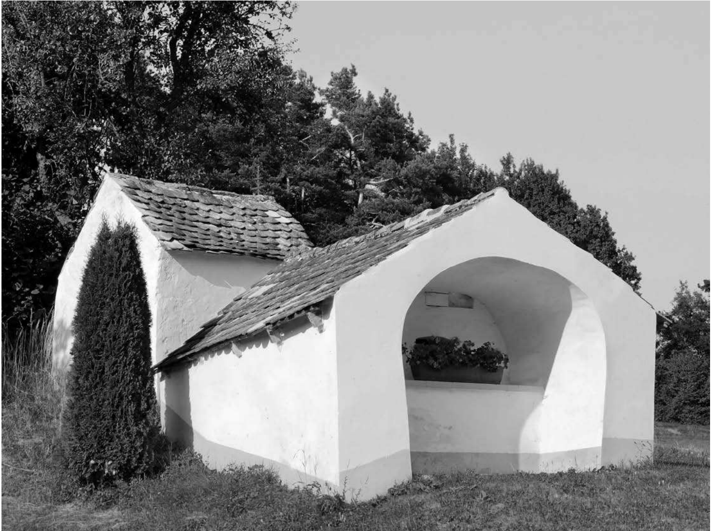
Backofen in Wolfersdorf
